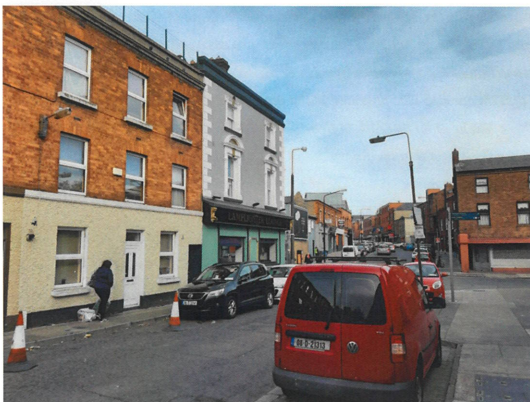
View on Brabazon Street elevation. The Referrers house is on the left, marked by the vertical poles above the parapet erected by the Referrer to enclose a roof garden created at that level since occupation.
