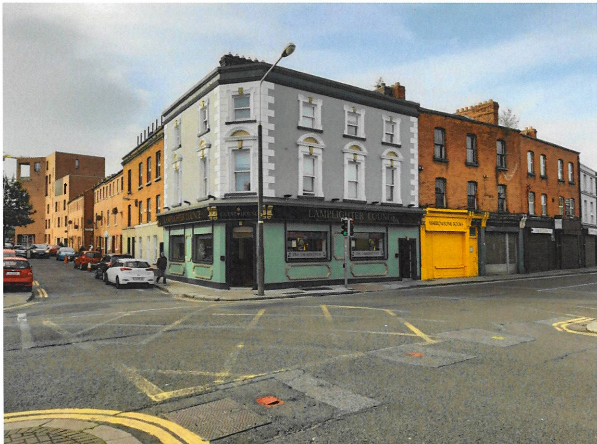
The Lamplighter building marks the corner in the Coombe and has been fully refurbished for its original use.
